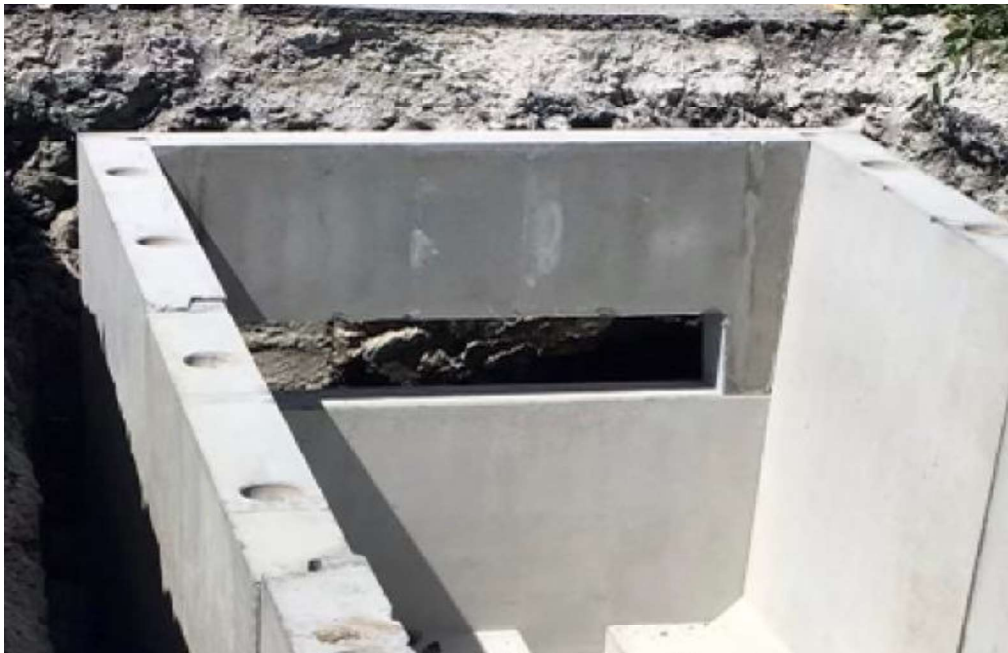
Figure 3 - Typical Joint Bay under construction (pre-cast)
