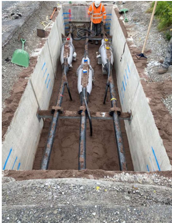
Figure 10 - Typical Joint Bay Backfilling Procedure
