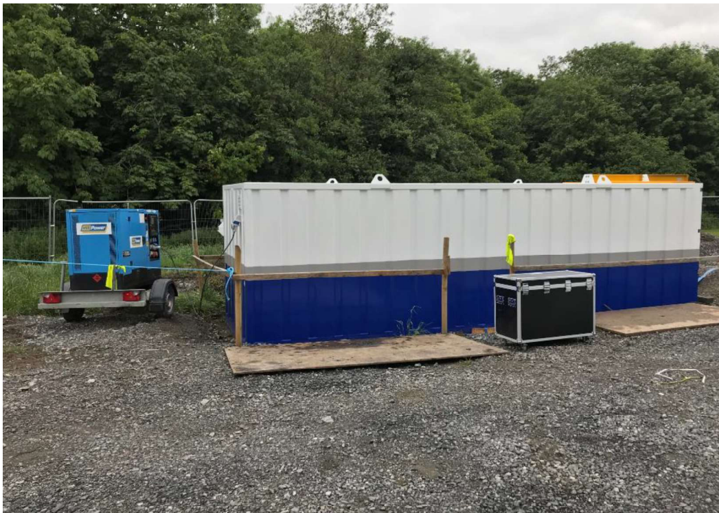
Figure 8 - Typical HV Cable Jointing Container
