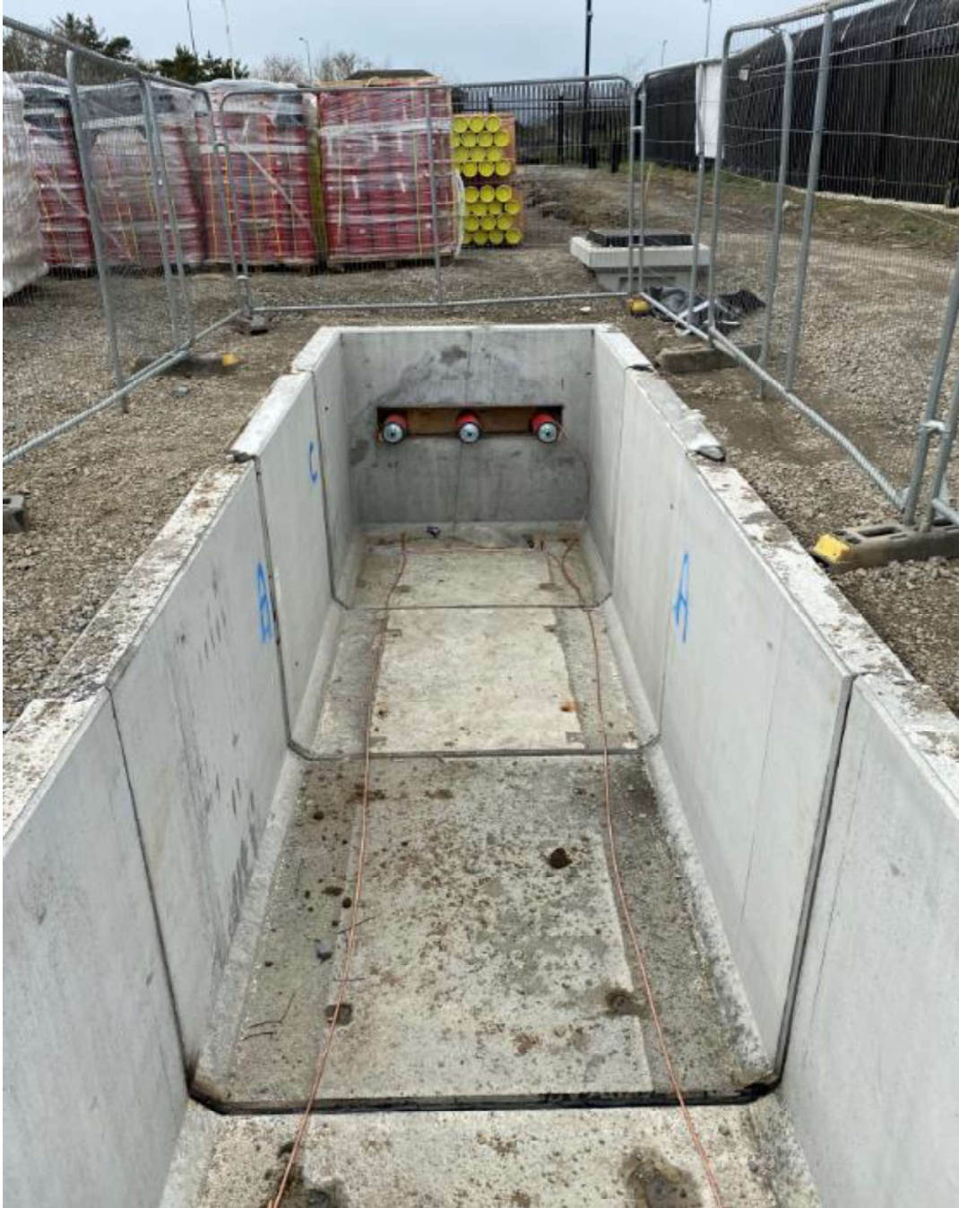
Figure 4 - Completed Joint Bay prior to Cable Installation (pre-cast)
