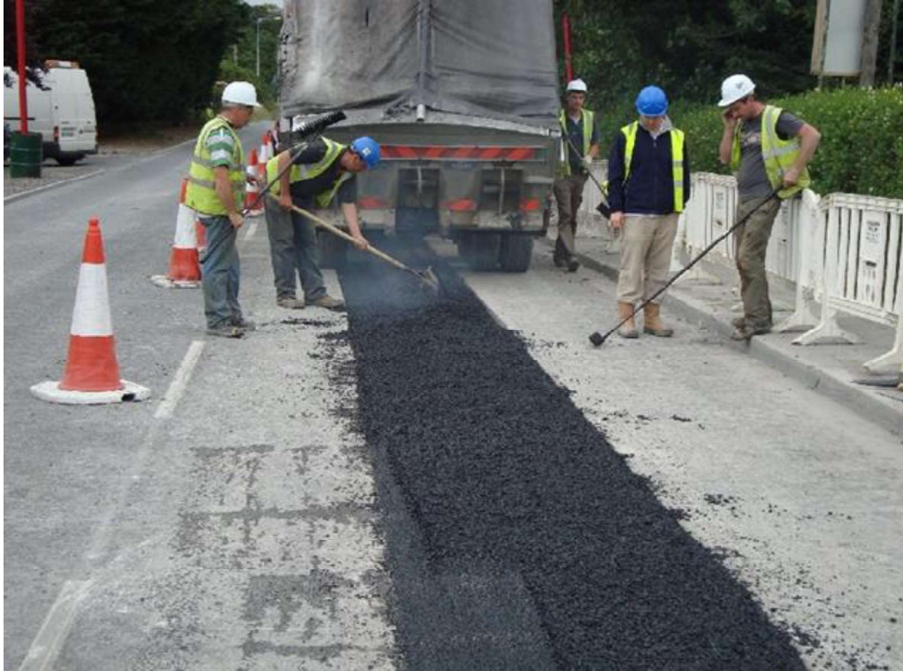
Figure 2 - Reinstatement of Road Surface Over Trench
