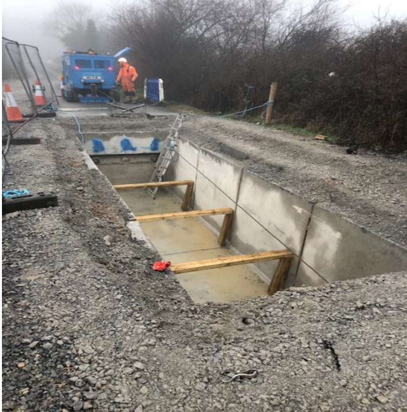
Figure 7 - Typical Winch Set Up for HV Cable Pulling Procedure
