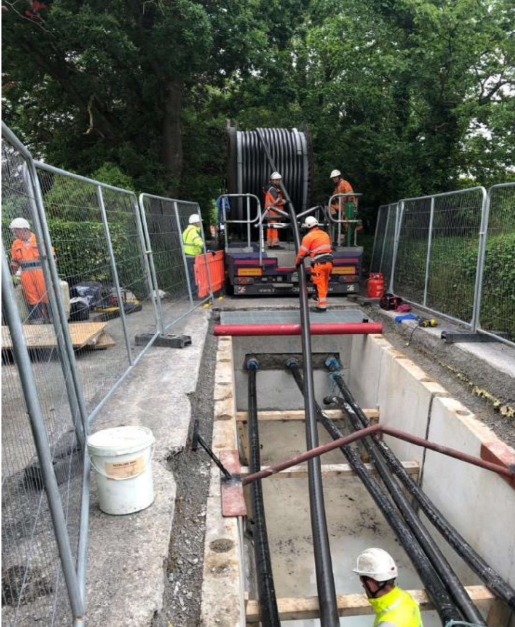
Figure 5 - Typical Set-Up of HV Cable Pulling Procedure
